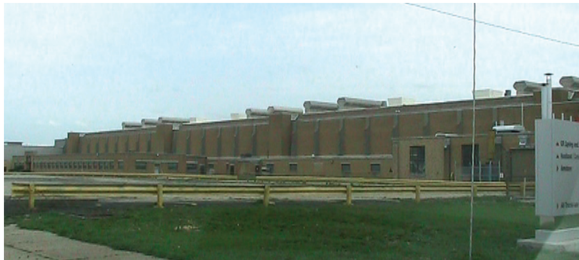
The Hangar42 facility was the subject of a suspicious land deal that led to felony charges.
